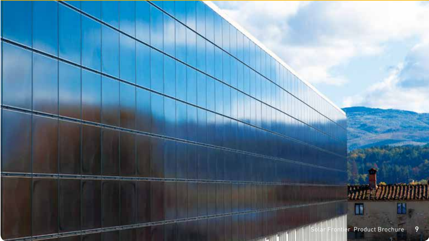
Bibbiena Facade Installation, 63 kW, Italy - Baraclit
