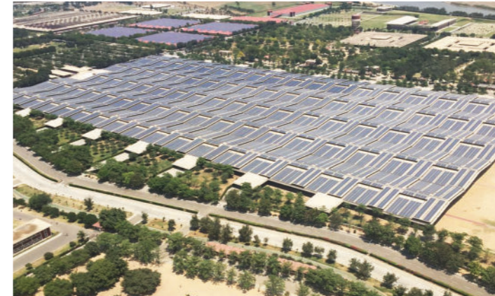
One of the largest Rooftop Solar Plants in the world at R.S.S.B Educational & Environmental Society
