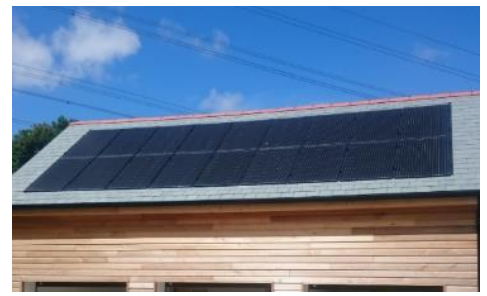
In-roof Mounting System
